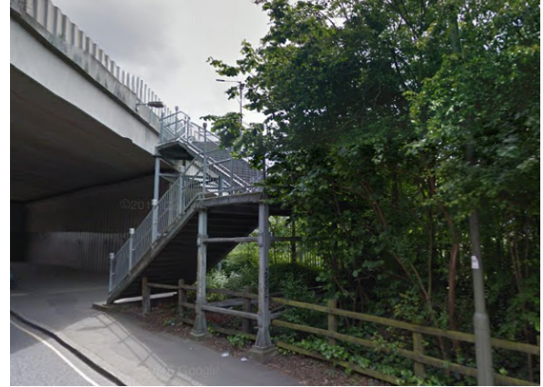
Figure 10: External stairs connecting Watford Way to Bunns Lane
