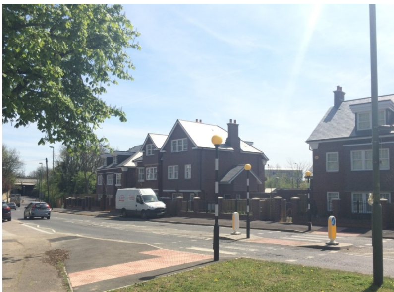
Figure 13: Churchill Place properties fronting Bunns Lane
